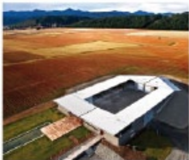
Winegrowers of Ara, Marlborough, New Zealand. The winery operations centre, known as 'The Dart' features a ZINCALUME® steel roof that folds down and over to shelter the courtyard from the prevailing winds.
